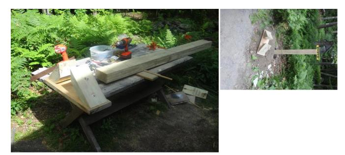
Cut a section of 2x8 to match the width of the Little Free Library. This is the base that rests on top of the post.
