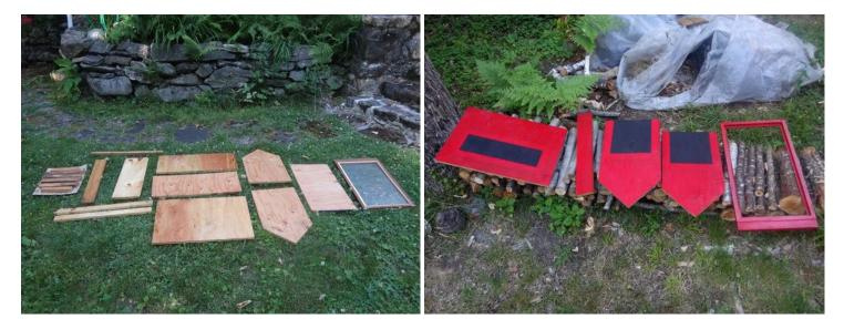
Paint all the interior surfaces with your favorite waterproof sealer. I used a translucent oil stain that I h ad on hand. Each joint will be glued as well as screwed, so for best glue adhesion avoid painting the s urfaces where the glue will be applied.
