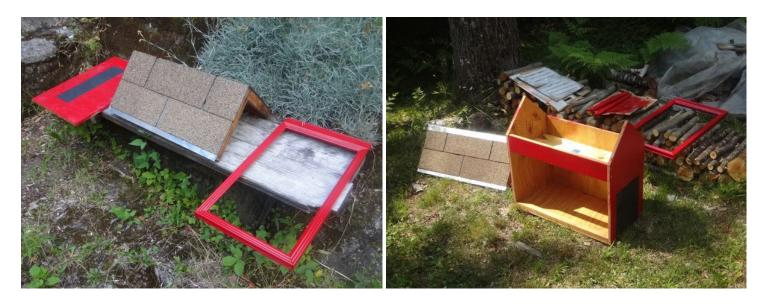
Apply wood glue and screw the brace and trim pieces to the plywood roof. Cut the flashing and roofin g shingles to fit. Nail or staple them in place.
